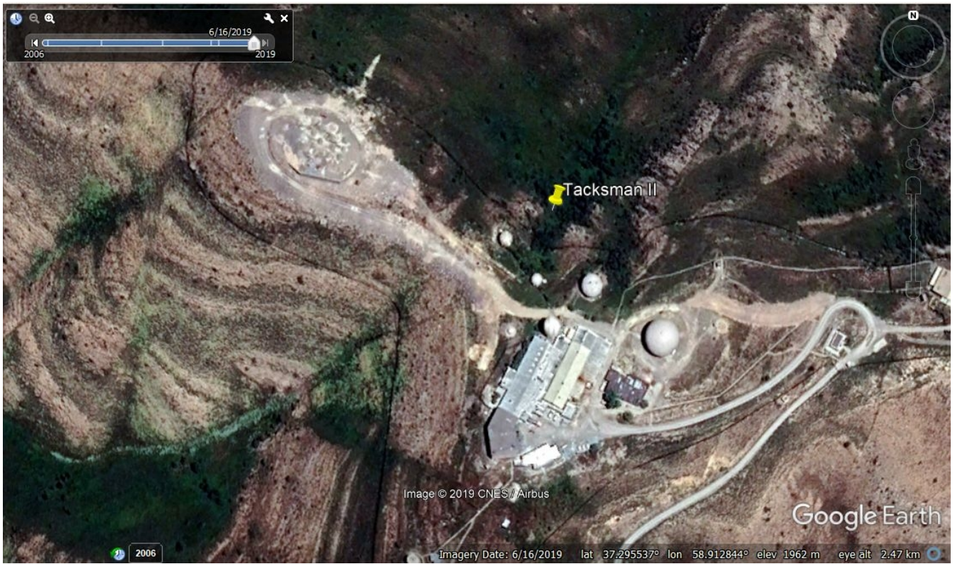
New Construction at TACKSMAN II June 2019
