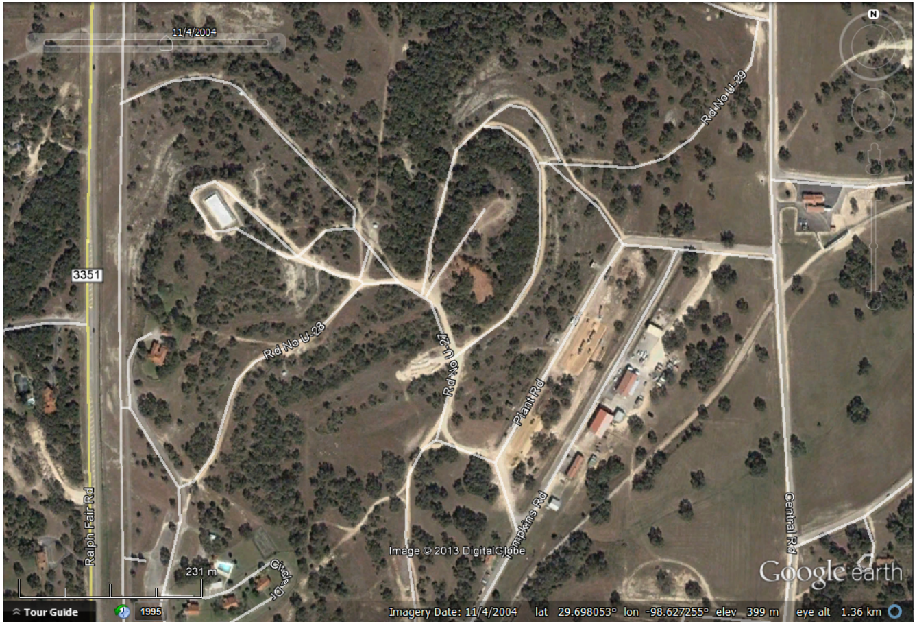
Beginning of construction between Tompkins and Plant Rds, 2004-11-04
