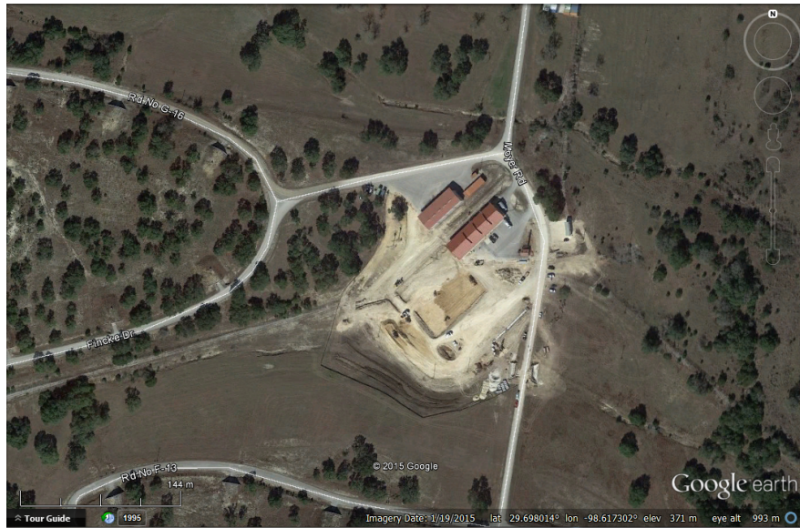
New large building under construction, 2015-01-19
