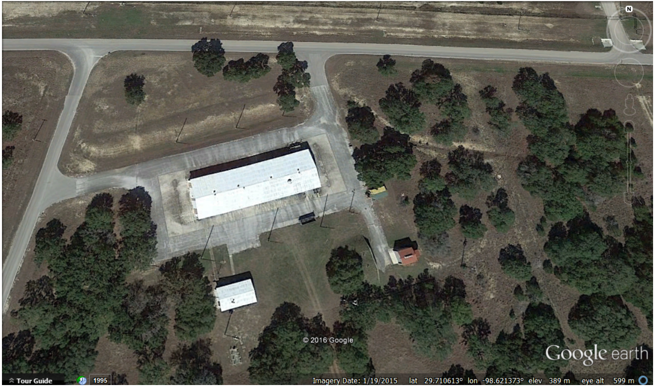
Possible explosives warehouse, 2015-01-19. Note the three tall masts along the north and south sides of the building.
