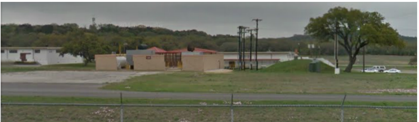
Google Street View image of generator enclosure and bunker as seen from Ralph Fair Road. Image date given as March 2011
