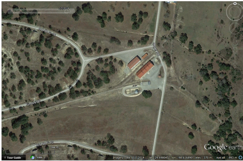
Area of new construction, 2014-02-07
