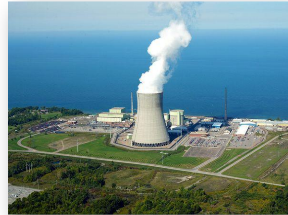
Nine Mile Point ~ Courtesy Constellation Energy
