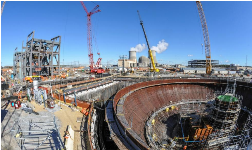
Construction of Vogtle Unit 3, January 2014 ©Georgia Power Company
