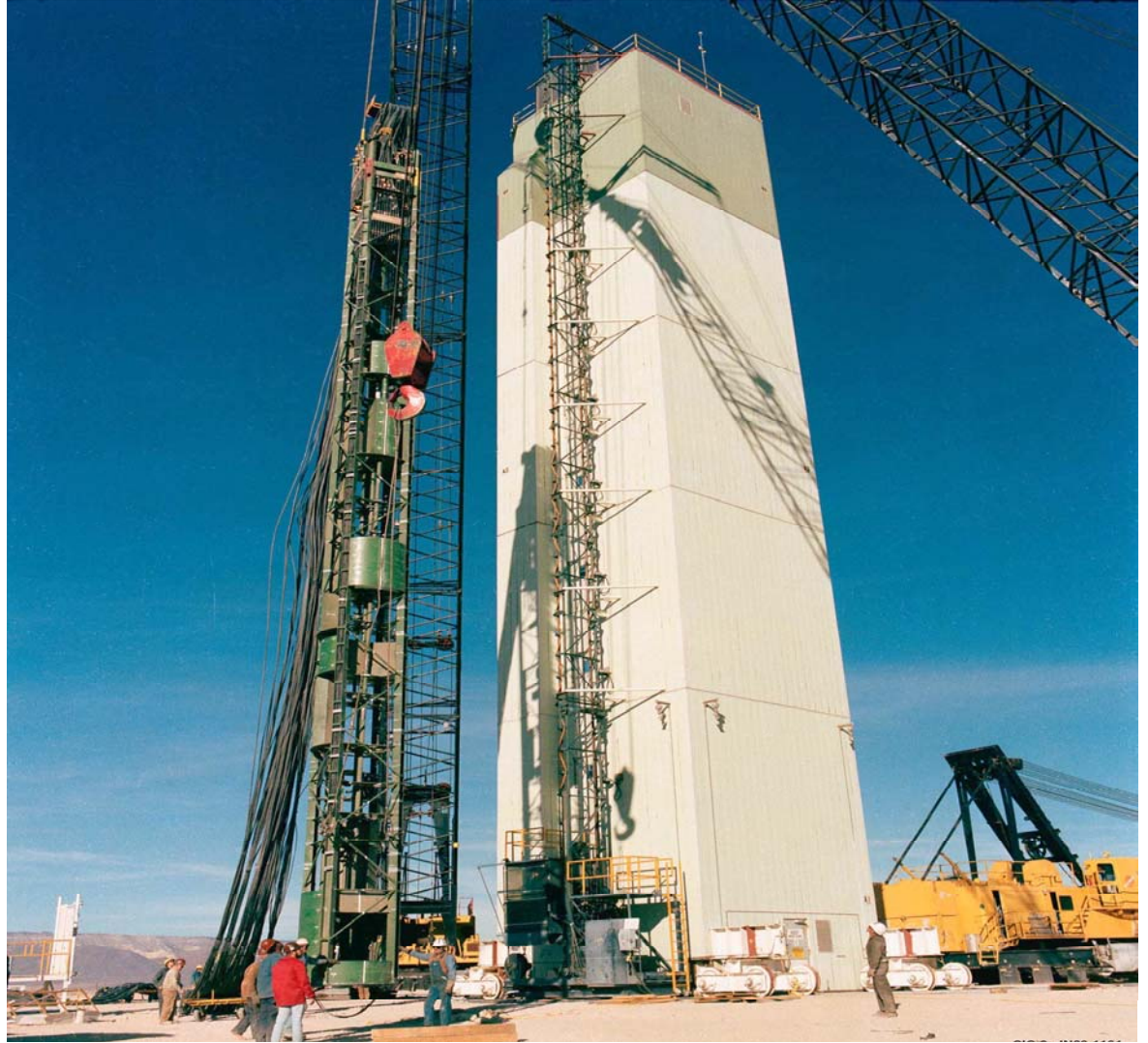
Figure 3-3. Close-up shot of tower housing test rack prior to device emplacement. Photo courtesy Los Alamos National Laboratory.
