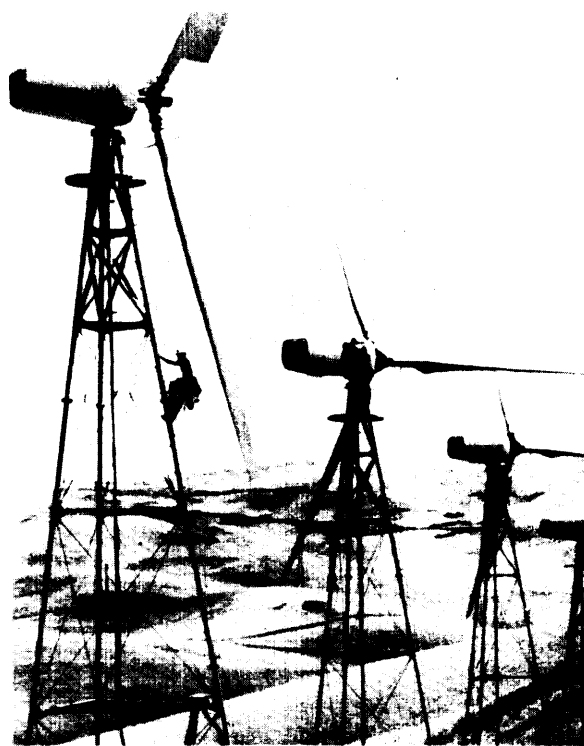
Small U.S.-made wind turbines.
