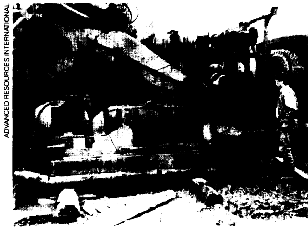
Truck-mounted drilling rig used for oil well drilling at Langepas, Western Siberia.
