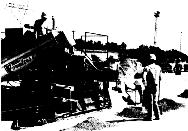
Photo credit: American Public Works Association
