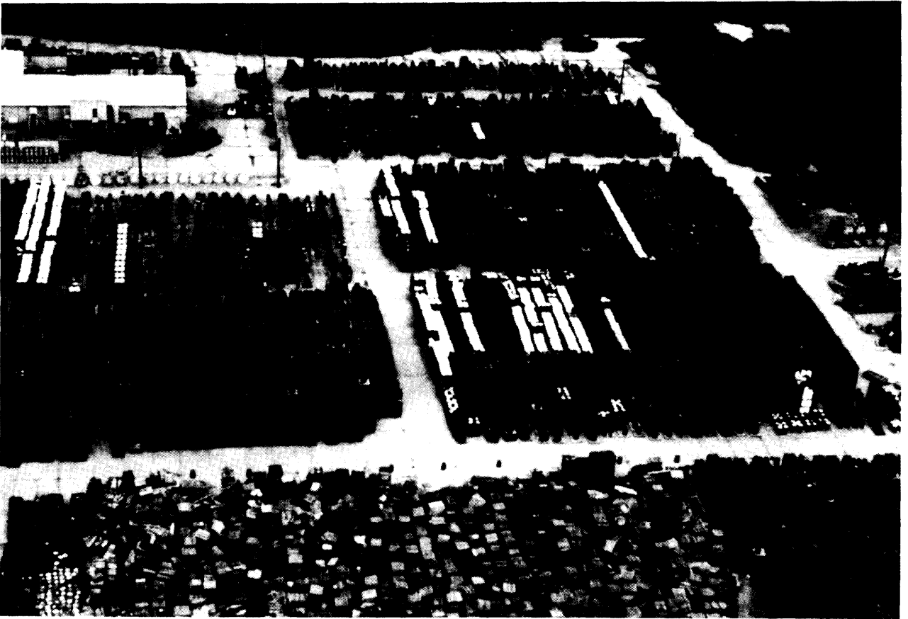
Photo credit: U.S. Department of Energy
