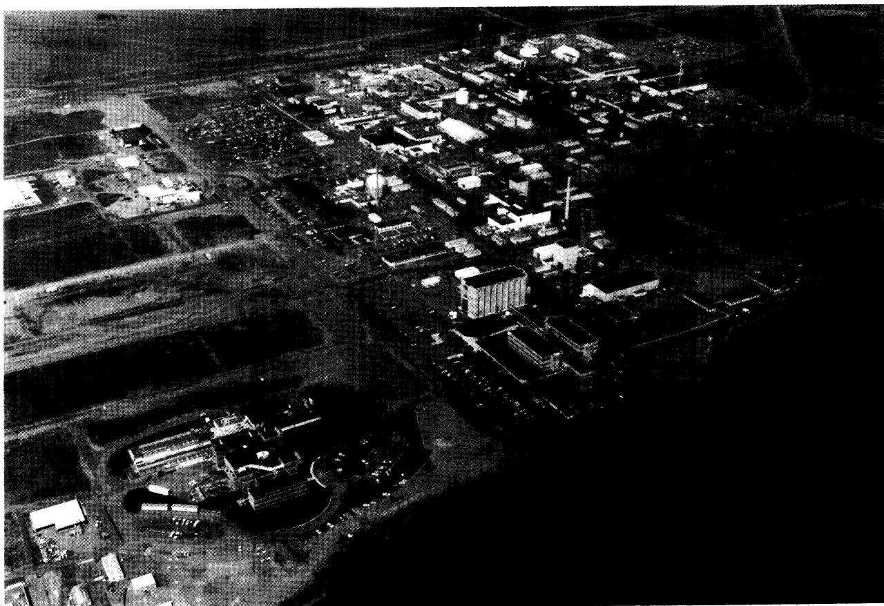
Photo credit: U.S. Department of Energy
