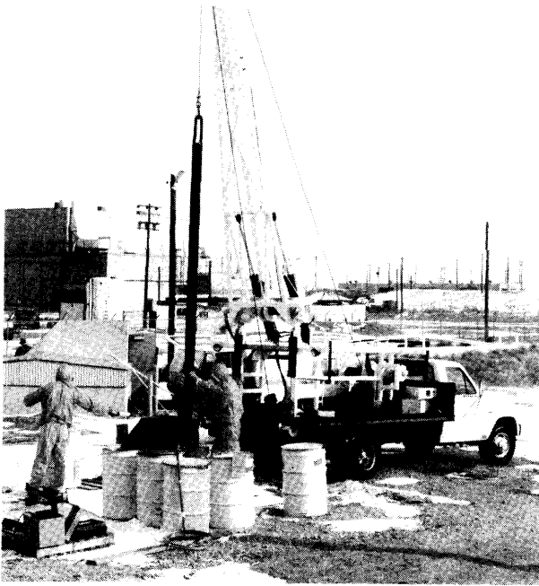
Photo credit: U.S. Department of Energy
