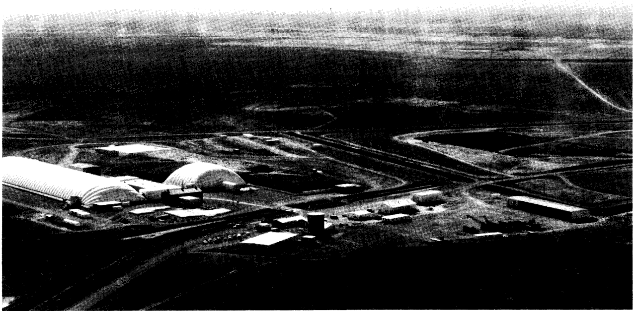
Photo credit: U.S. Department of Energy
