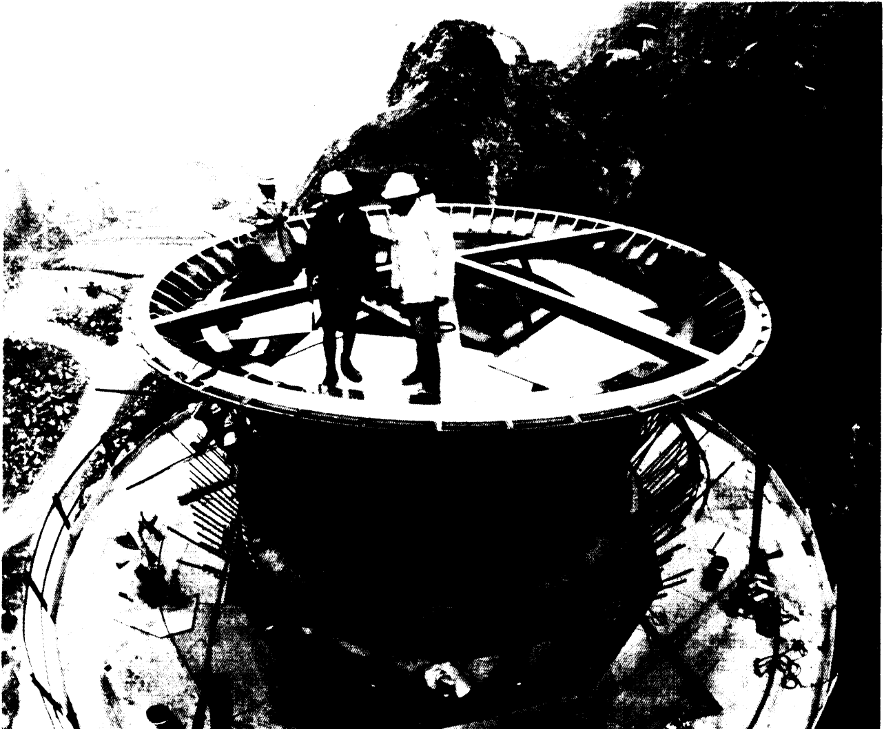
Photo credit: Bechtel Power Corp.
