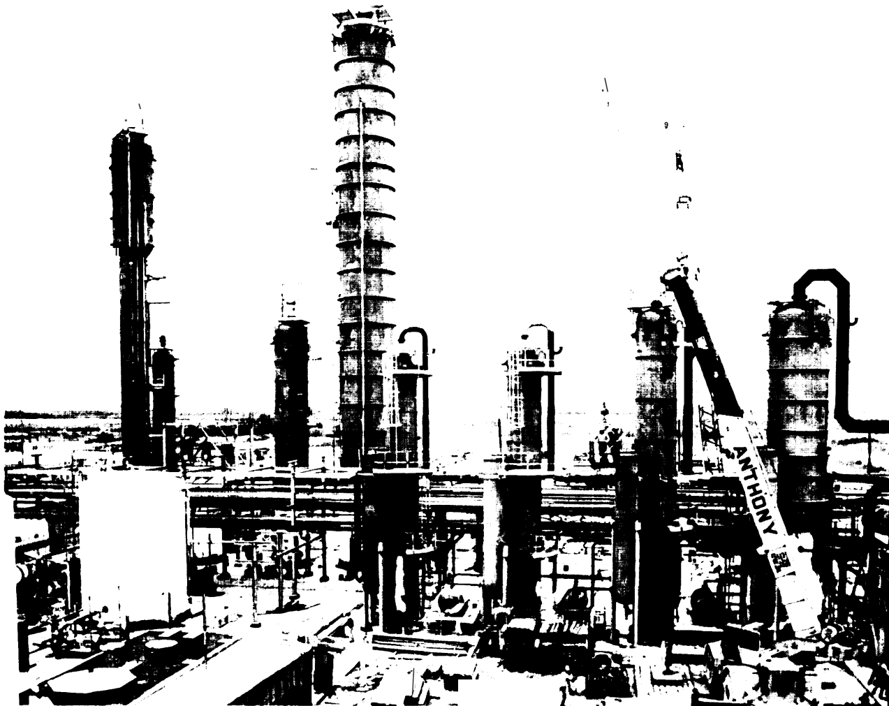
Photo credit: PPG Industries, Inc
