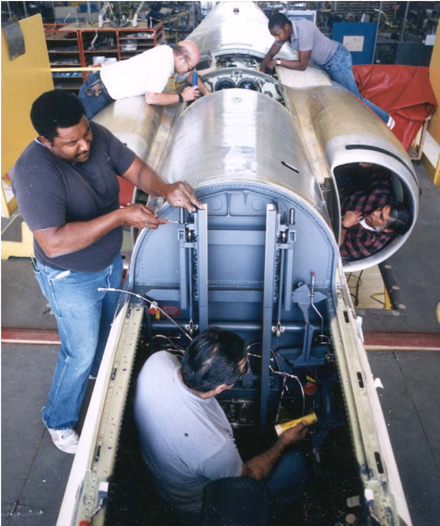
Lockheed workers build a new version of the U-2, now redesignated TR-1. (Lockheed Martin)
