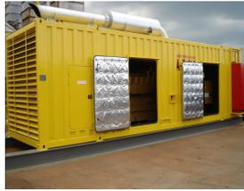
**Typical external appearance of a transportable diesel generator set.**
