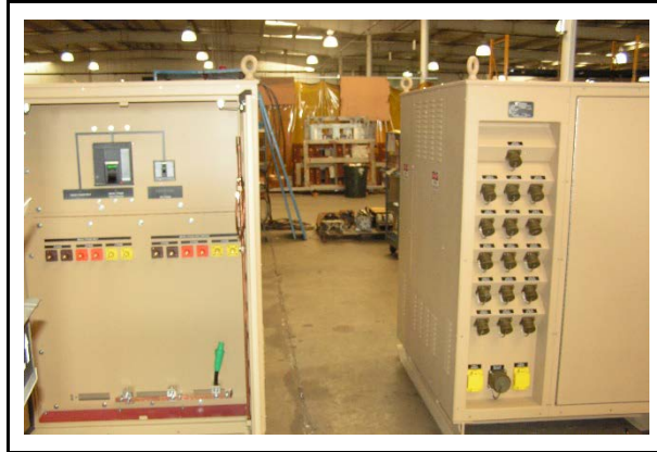
Figure E-9. Secondary distribution center
